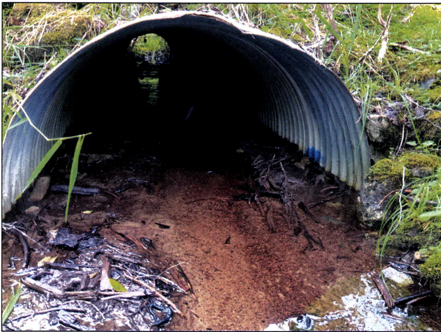
Figure 3.—Culvert at waypoint 1256.
