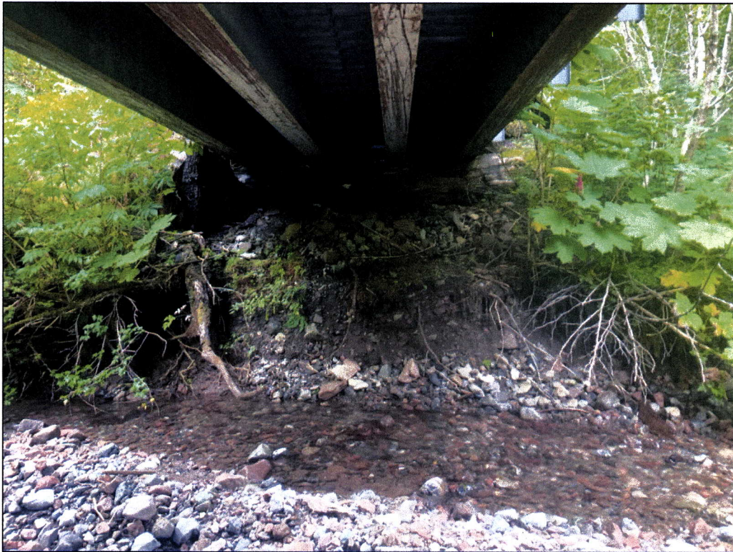
Figure 2.—Bridge abutment with some riprap eroded at waypoint 1469.
