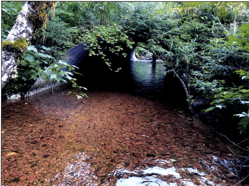
Figure 3.—Culvert at waypoint 1257.
