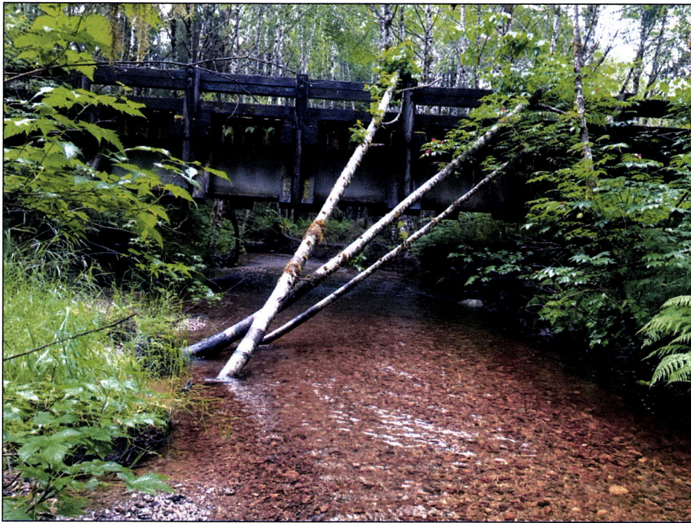
Figure 2.—Bridge at waypoint 1231.
