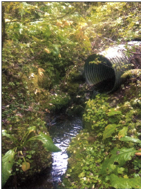
Figure 3.—Perched culvert outlet at waypoint 1825.
