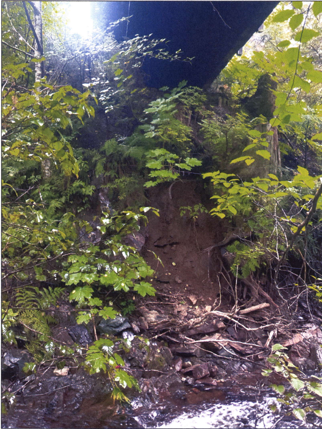
Figure 2.—Erosion on river-left embankment at waypoint 1630.
