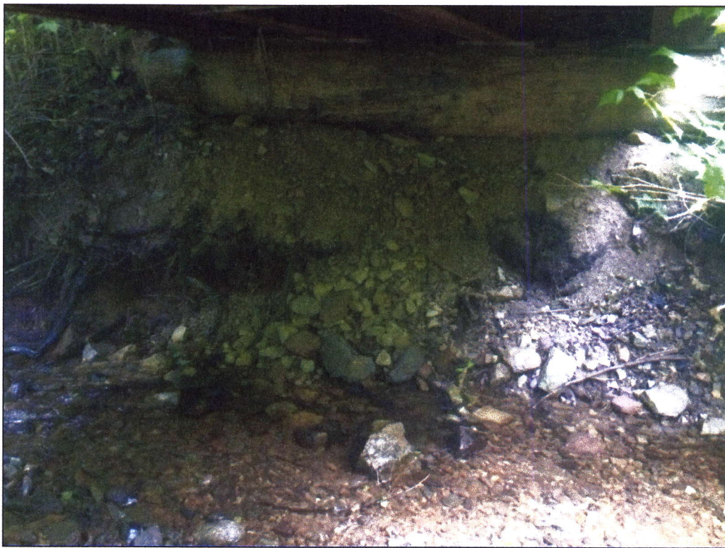
Figure 2.—Eroding river-right bridge abutment at waypoint 2279.
