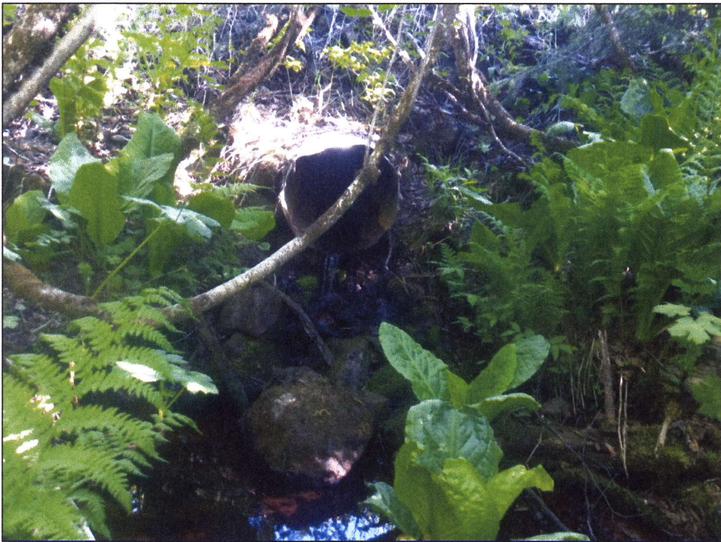
Figure 4.—Perched culvert outlet at waypoint 405.
