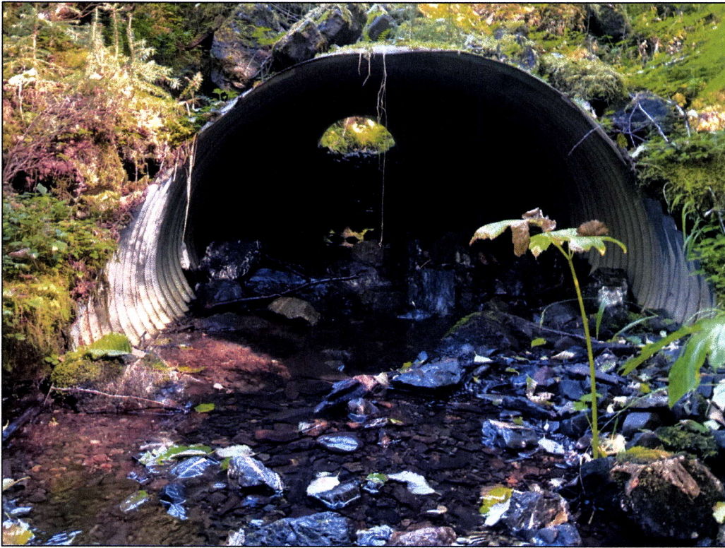
Figure 2.—Culvert outlet at waypoint 1557.
