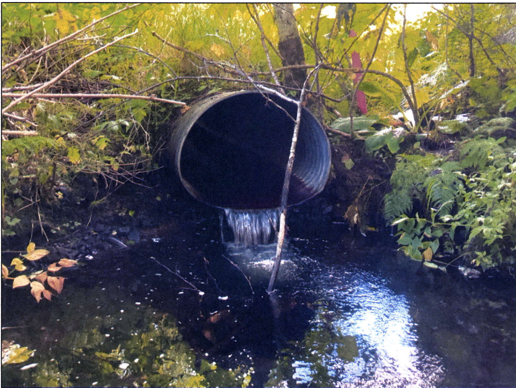
Figure 2.—Perched culvert outlet at waypoint 1561.
