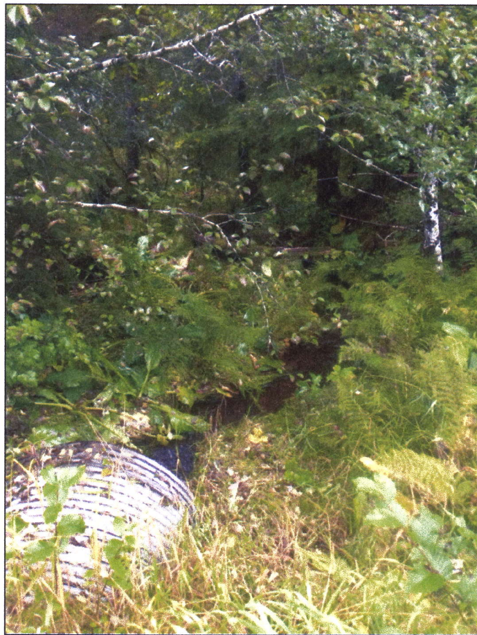
Figure 2.—Culvert outlet at waypoint 2434.
