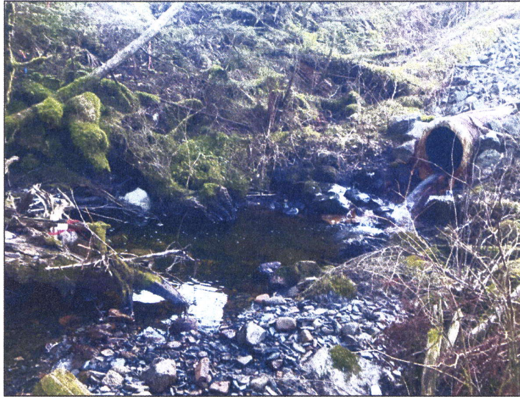
Figure 1.—Perched culvert outlet and pool at waypoint 1068.
