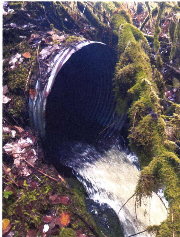
Figure 3.—Perched culvert outlet at waypoint 1036.
