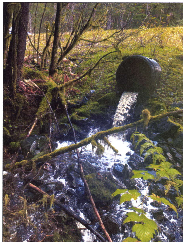
Figure 3.—Perched culvert outlet at waypoint 1030.
