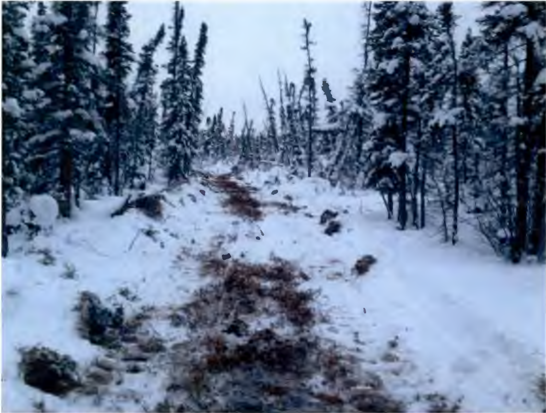
Figure B3. Results of one pass with roller chopper while snow is still around 18"
