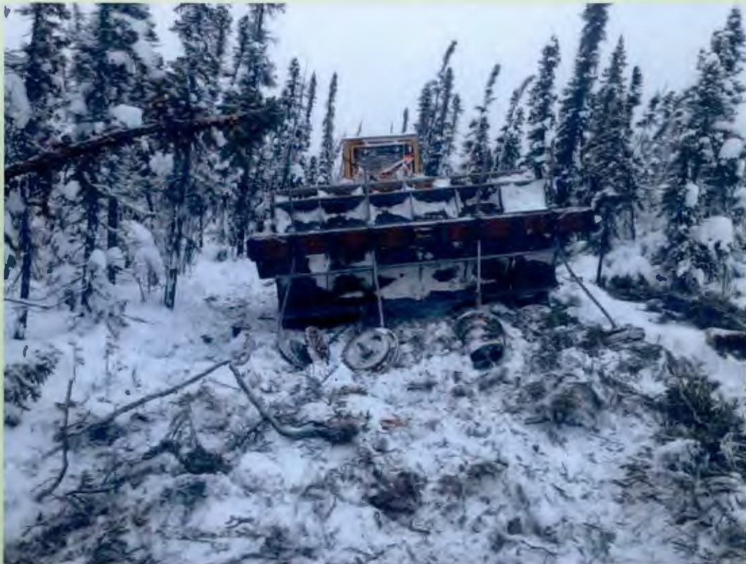
Roller Chopper with scarification discs in 18+” of snow Dec 2013
