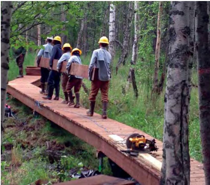
Great Land Trust partnered with the Student Conservation Association to build a light penetrating wetland boardwalk that provides an easy way for people to experience the Palmer Hay Flats Game Refuge. Kim Sollien/Great Land Trust
