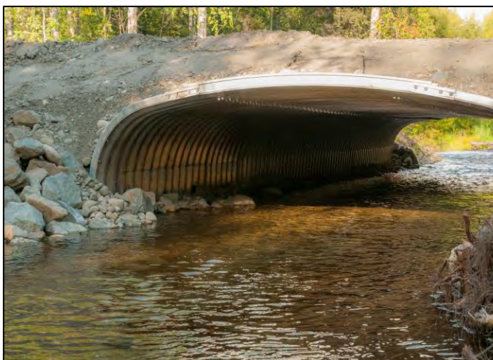
Figure 21. Fish passage culvert installed on Caswell Lake Road in 2014.
