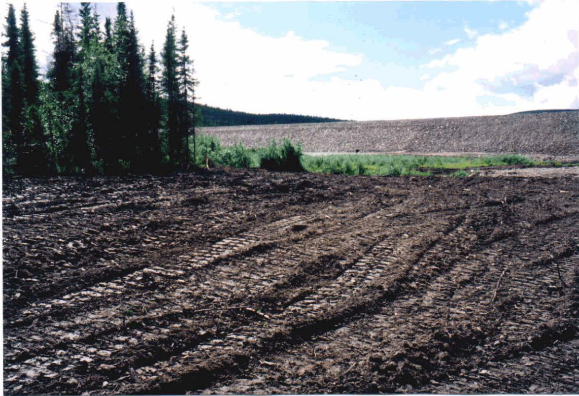
Figure 2. The construction zone adjacent to the catchment basin was regraded and with the natural moisture, fines, and organic materials present, natural revegetation should occur rapidly (top and bottom photos, July 1996).
