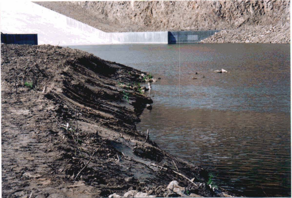
Figure 3. The completed spillway and the upper portion of the catchment basin (top photo) and the constructed outlet channel connecting the catchment basin with Fish Creek (bottom photo) will provide fish passage.
