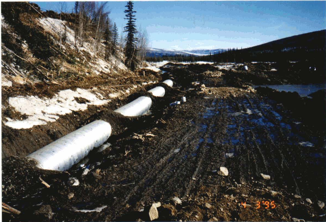
Figure 5. A culvert was placed in the diversion ditch on the north side of the valley to move Fish Creek through the construction zone (top photo). Stripping of overburden at the freshwater dam began in late March 1995 (bottom photo).
