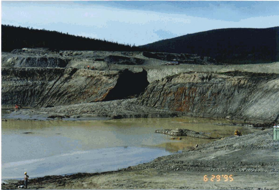
Figure 8. The freshwater dam excavation was flooded on June 29 (top photo). Most of the water had been removed by July 5 and equipment was working to clean up the excavation (bottom photo).
