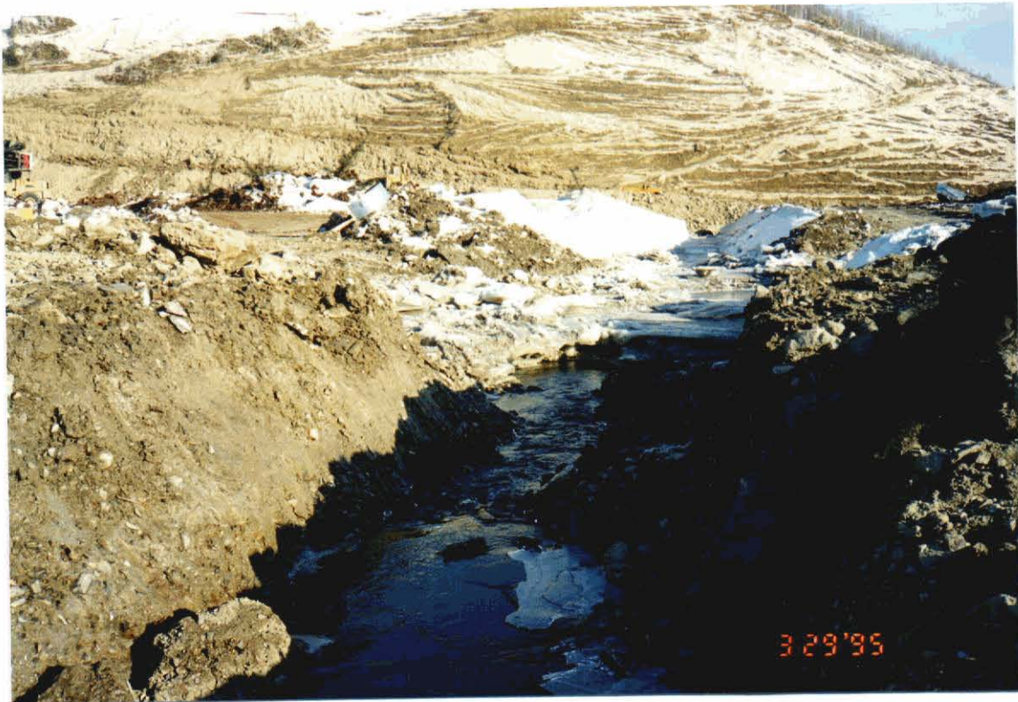
Figure 6. A channel plug was placed in Fish Creek but not completely removed (top photo). On April 3, 1995, when the site was rechecked the channel had been cleaned and the plug removed (bottom photo).
