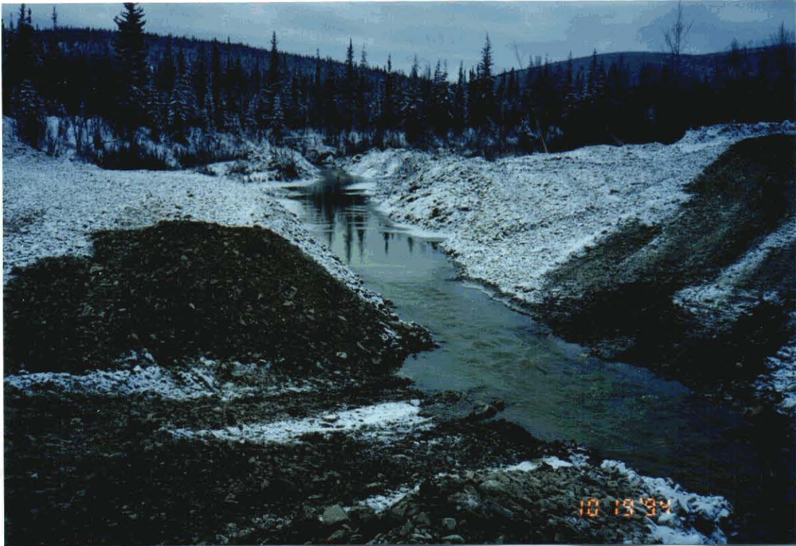
Figure 4. The diversion ditch upstream of the freshwater dam (top photo) and the diversion ditch through the construction zone (bottom photo) in October 1994.
