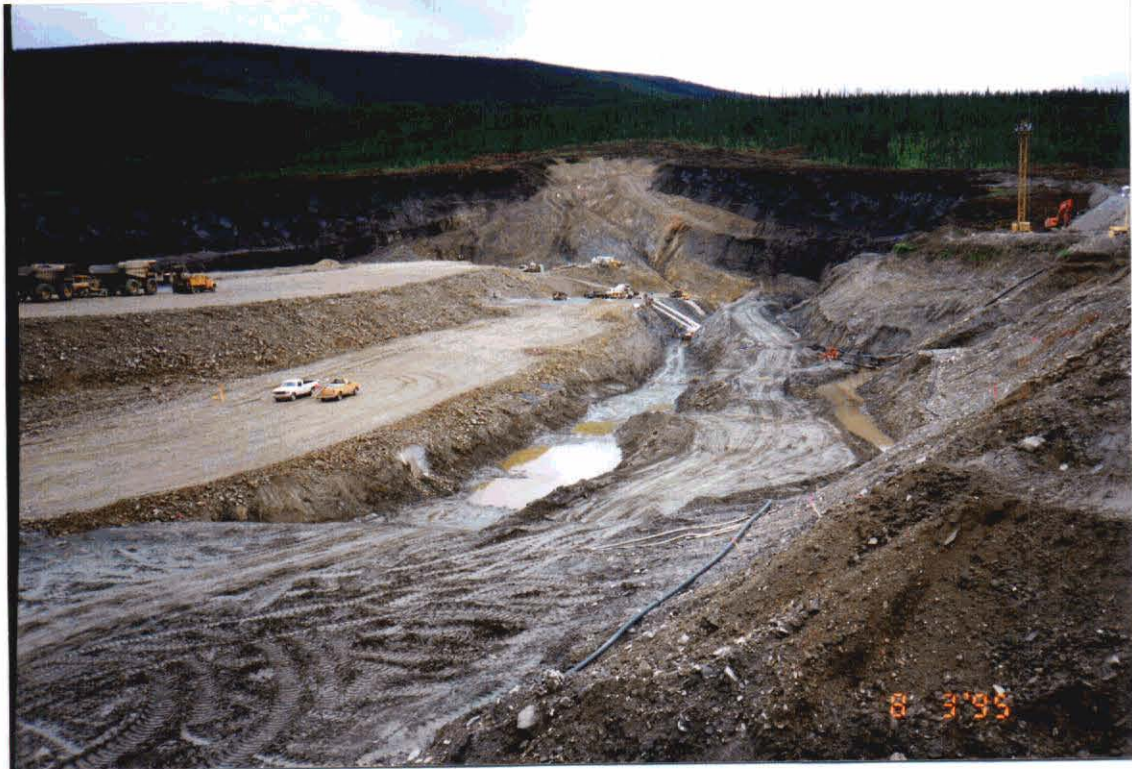
Figure 10. Backfilling using select and random fill material to build the freshwater dam was in progress (top photo). Freshwater dam nearly complete in early October 1995, viewed from the hills overlooking the Fish Creek valley (bottom photo).
