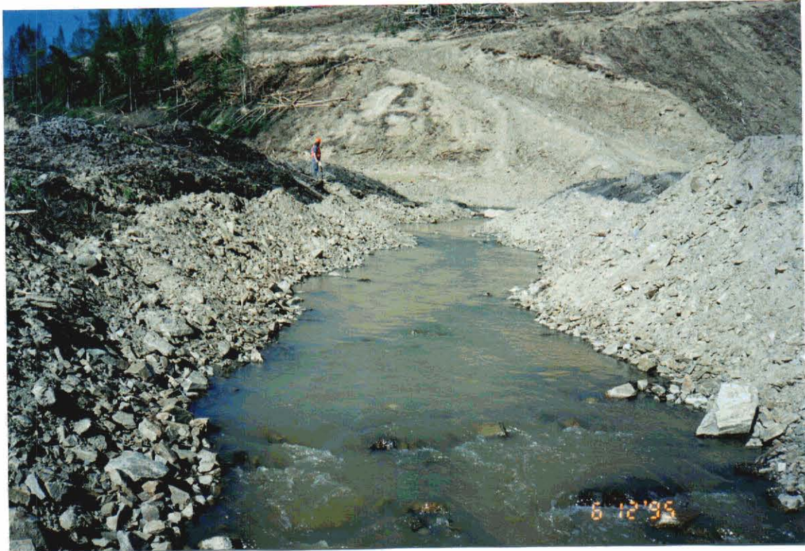
Figure 7. The diversion channel through the freshwater dam construction zone had been stabilized (top photo). Excavation for the freshwater dam and pumping of water from the excavation continued (bottom photo).
