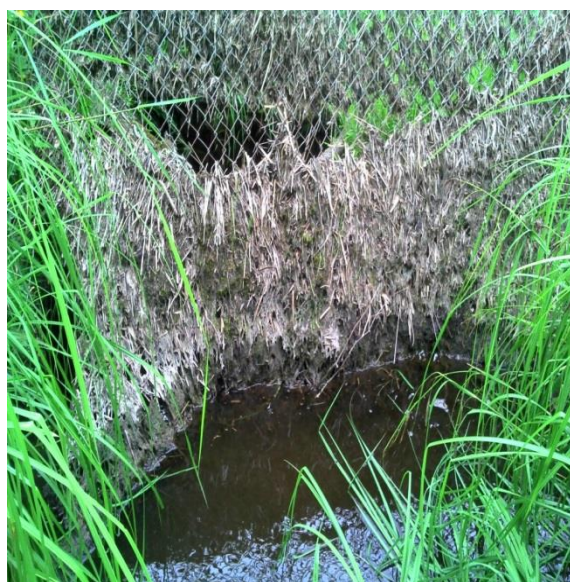
Figure 2.—Chain link fence clogged with debris around airport.
