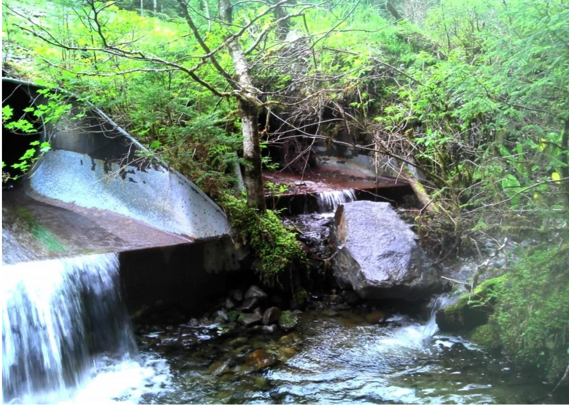
Figure 1.—Double culverts outlets under Mitkof Highway.
