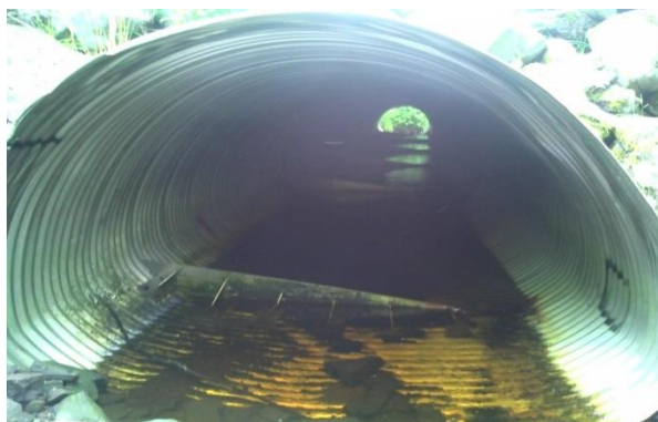
Figure 2.–Bafled culvert under Mitkof Hwy.
