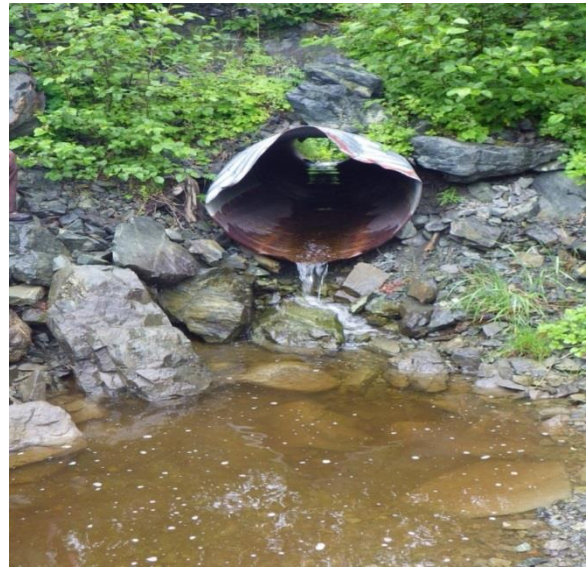
Figure 2.–Perched and damaged culvert near mouth of Cannery Creek (WPT# 3)
