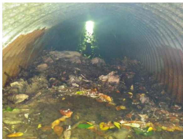
Figure 2.–16.9 Mile Creek culvert inlet below the Haines Highway with large debris mound that creates a 2ft drop.
