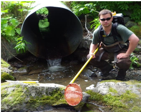
Figure 1.–Rick Hoffman stands in front of perched culvert below Mud Bay Road.
