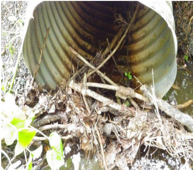
Figure 1.–Culvert filled with debris, restricting flow (WPT# 7).
