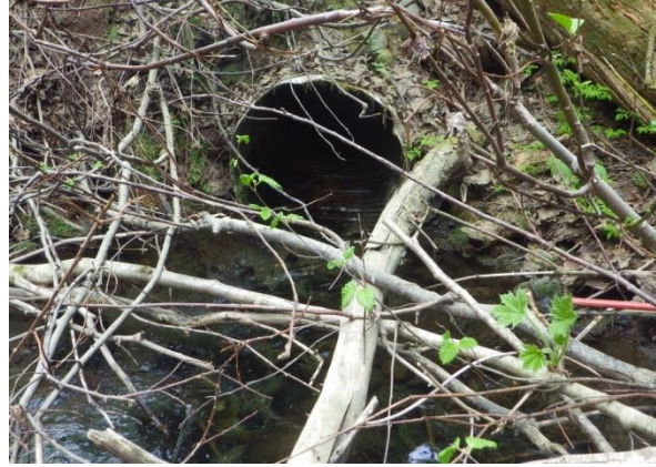
Figure 2.—Culvert under overgrown road.
