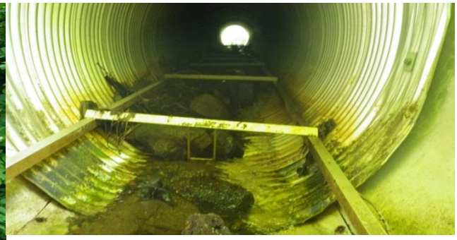
Figure 2.–Culvert beneath Mud Bay Road with fish passage modifications.
