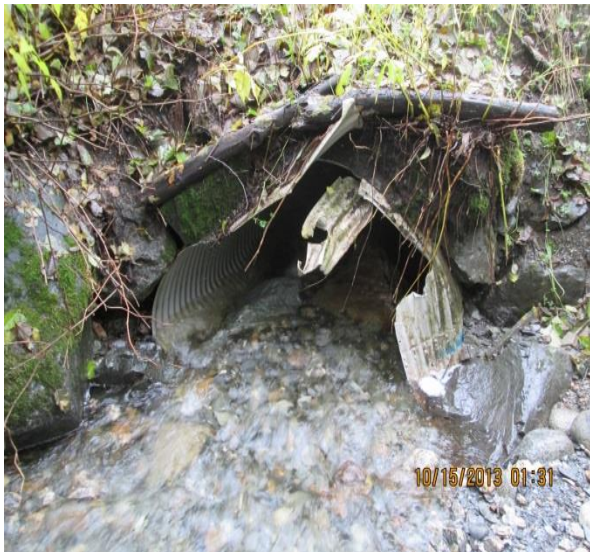
Figure 1.–Mangled culvert in Switzer Village.
