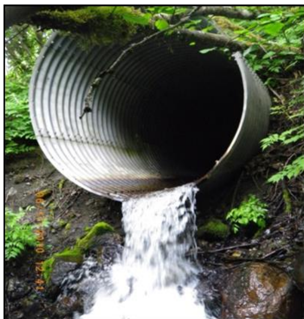
Figure 1.–Perched culvert on Falls Creek.
