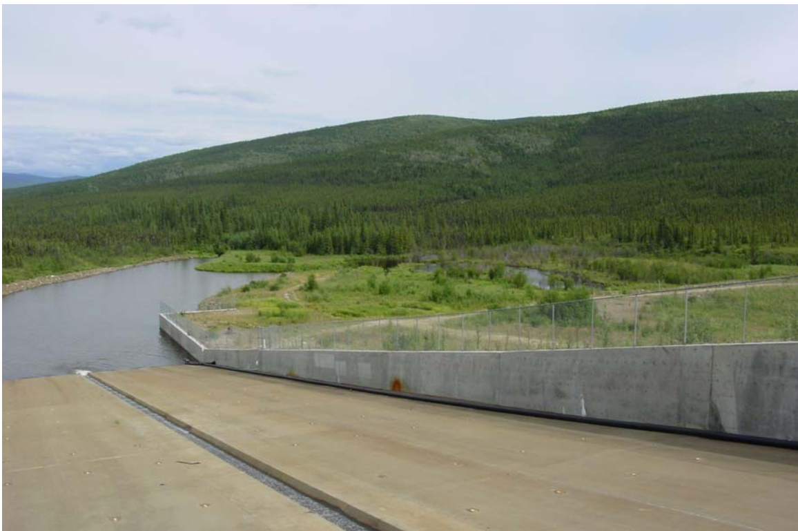
Figure 10. Spillway in Ft. Knox freshwater dam (August 2006).
