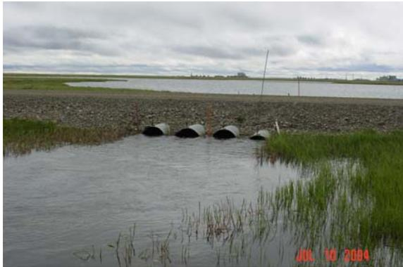
**FC1 Crossing**– View of downstream side of culvert battery, all culverts are more than 50% submerged.
