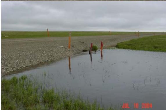
**FC1 Crossing**- View of upstream side of culvert battery, culvert inlets are completely submerged.
