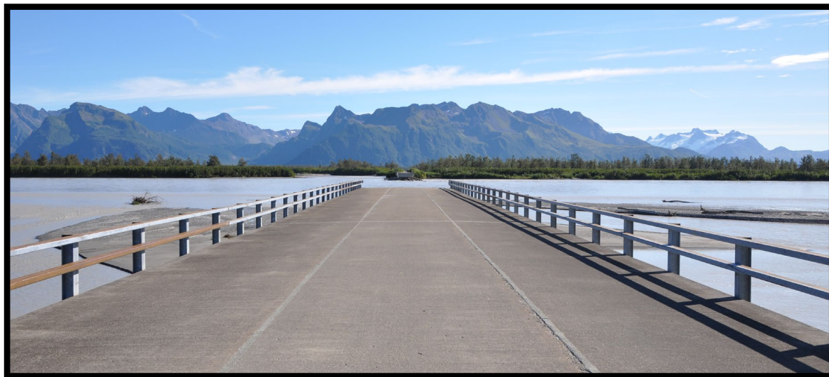
Washed out bridge at mile 36. Often called "36 Mile Bridge."
