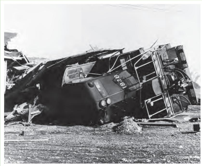
*Above: A 200 ton diesel switch engine of the Alaska Railroad lies on its side more than 200 feet from its original position in Seward, Alaska, following the Alaska Earthquake and tidal wave 3/27/64.*
