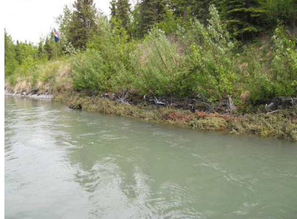
Figure 13. This combination project (rootwads plus cabled spruce trees) provides bank protection and a diversity of habitat cover along the bank (left bank near river mile 31).
