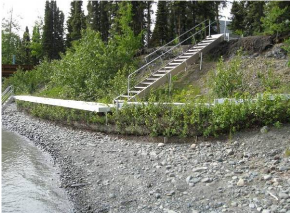
Typical bioengineered bank
