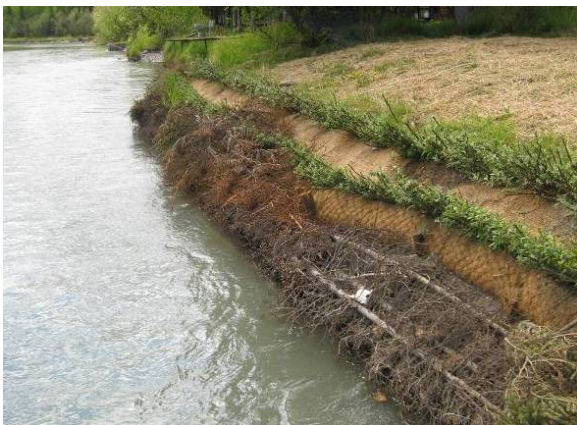
Typical combination approach (cabled spruce trees and bioengineered bank)
