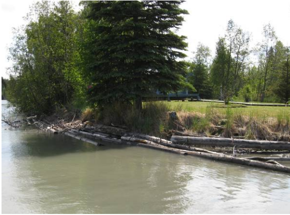
Typical tethered log treatment
