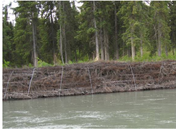
Large cabled spruce tree revetment with multiple stacked layers
