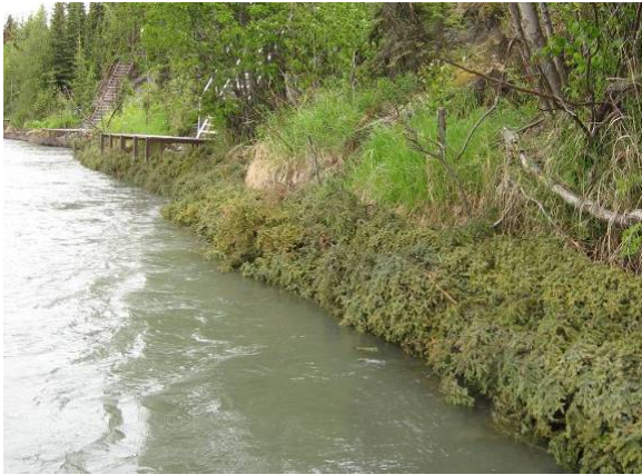
Typical cabled spruce tree revetment
