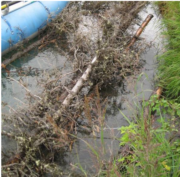
Figure 31. Loosely packed CSTs allow for juvenile salmon access to within and behind the structure, where there is good velocity refuge, overhanging vegetation, and access to undercut banks.
