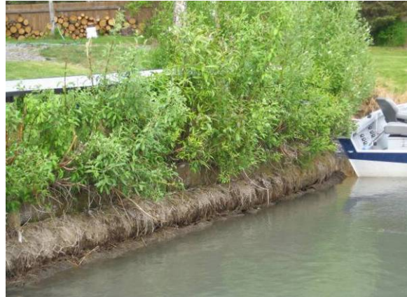
Bioengineered bank with coir log toe and good willow growth
