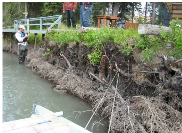
Combination approach using cabled spruce trees and rootwad revetment
