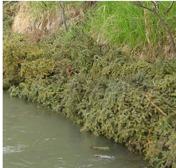
Figure 32. Tightly packed CSTs may provide more effective erosion control but may simplify the bank and limit access to within or behind the structure for juvenile salmon rearing.
