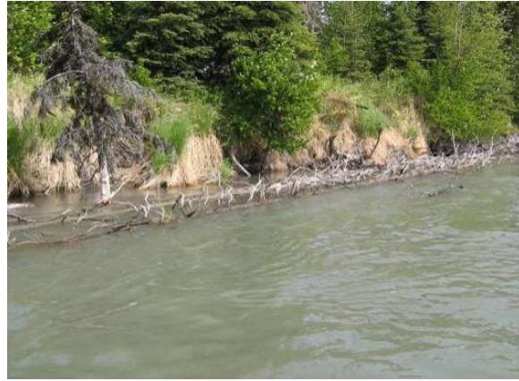
Typical tethered log treatment
