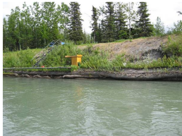
Figure 11. BEB near RM 31. BEB is halting erosion; however, fabric wraps are beginning to fail. Even with vigorous willow growth (as on the left side in this photo), eventual collapse of the wraps will undermine the bank and create continued erosion and failure of the willows.
