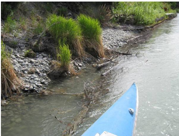
Figure 10. View looking upstream at BEB project near RM 31. Notice severe bank erosion and soil loss upstream of project (site of failed CST project) and effective bank protection provided by BEB.
