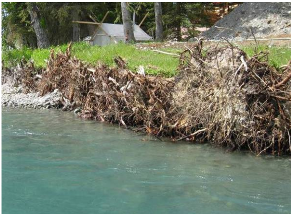
Typical rootwad revetment
