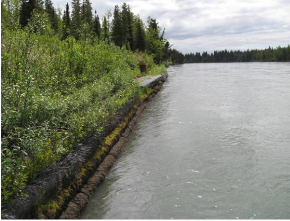
Figure 12. Bioengineered banks provide good bank protection but create linear, uniform banks with little cover habitat for juvenile fish (left bank near river mile 31).
