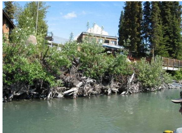
Rootwad revetment with willow live staking
