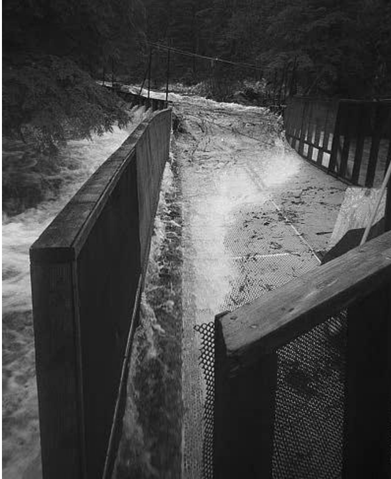
Figure 4.—View looking upstream on the dewatering table portion of the Slippery Creek smolt trap during moderately high flows. (note photograph is showing vertical panels constructed with plastic mesh which was changed prior to this reporting period to milled aluminum “smolt plate” identical to the flooring seen in the photograph).
