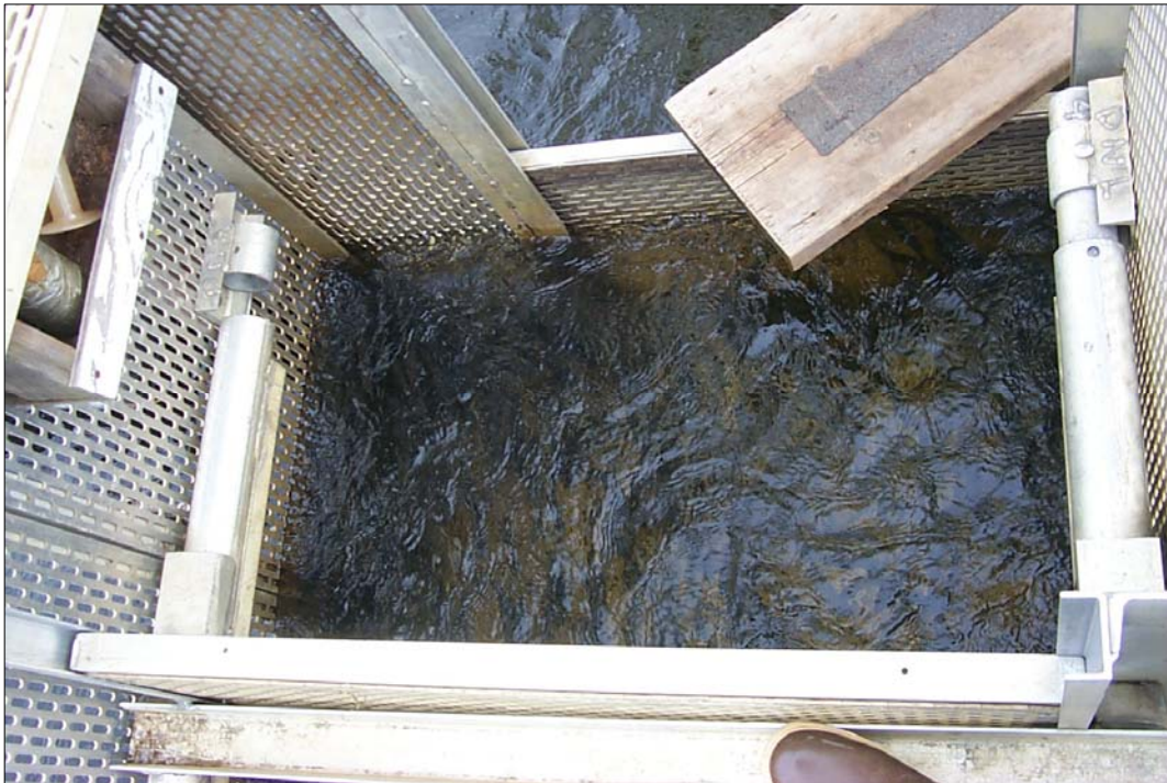
Figure 30. —Live box on Moose River weir. Note perforated metal panels and welded tube for crowder to slide on. Live box is about 10 x 4 ft, so crowder is used to concentrate fish in one end and then moveable panels are dropped in to hold them in small area for easy netting.
