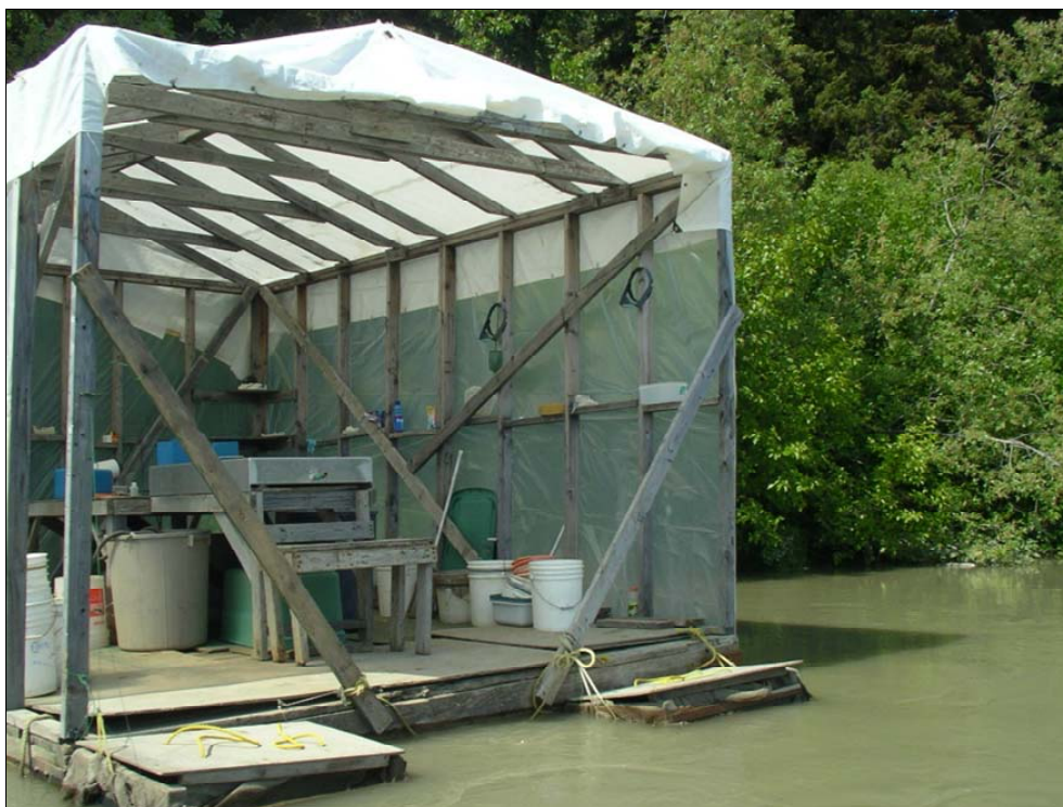
Figure 34. —Taku river floating tagging shed mounted on sealed steel drums. Note holding pens in front.
