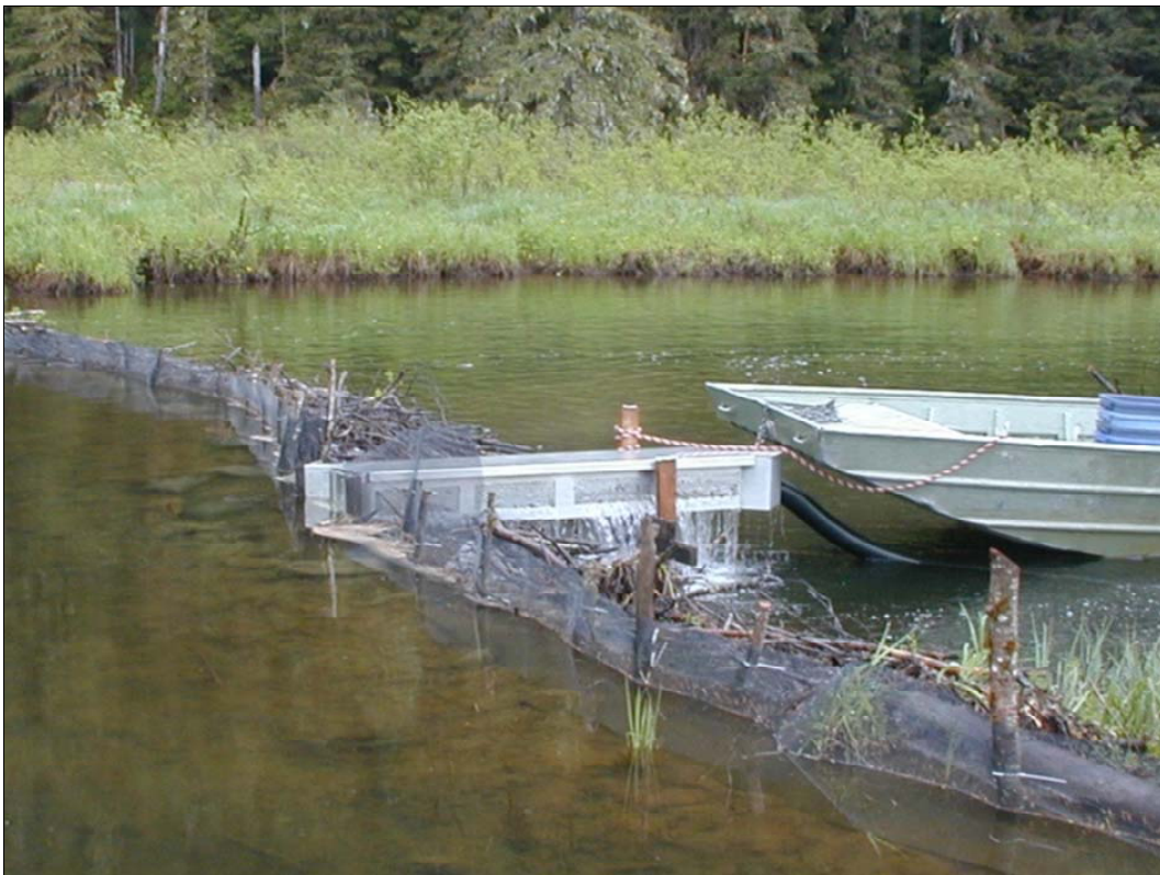
Figure 20. —The trough of a spill trap installed in a long beaver dam on a tributary of the Berners river. A mesh fence blocking many trickles should be installed in 6 to 12 in of water, upstream of the crest of the dam.
