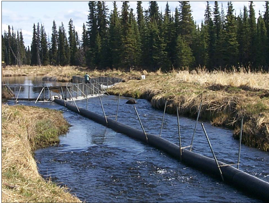
Figure 15. –Moose Creek smolt weir and culvert leading to live box. Note culvert must be staked down to keep it from being pushed downriver and separating at joints.
