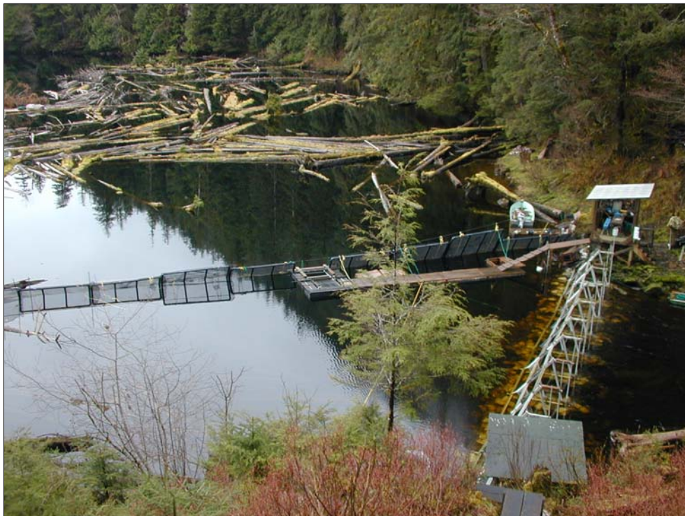
Figure 16. –The coho salmon smolt weir at the outlet of Hugh Smith Lake and the aluminum framework of the adult weir. The smolt weir is located in deeper water where the current is less severe. A cable provides support along the top. A floating walkway provides convenient access between the inclined plane trap and the tagging operation.
