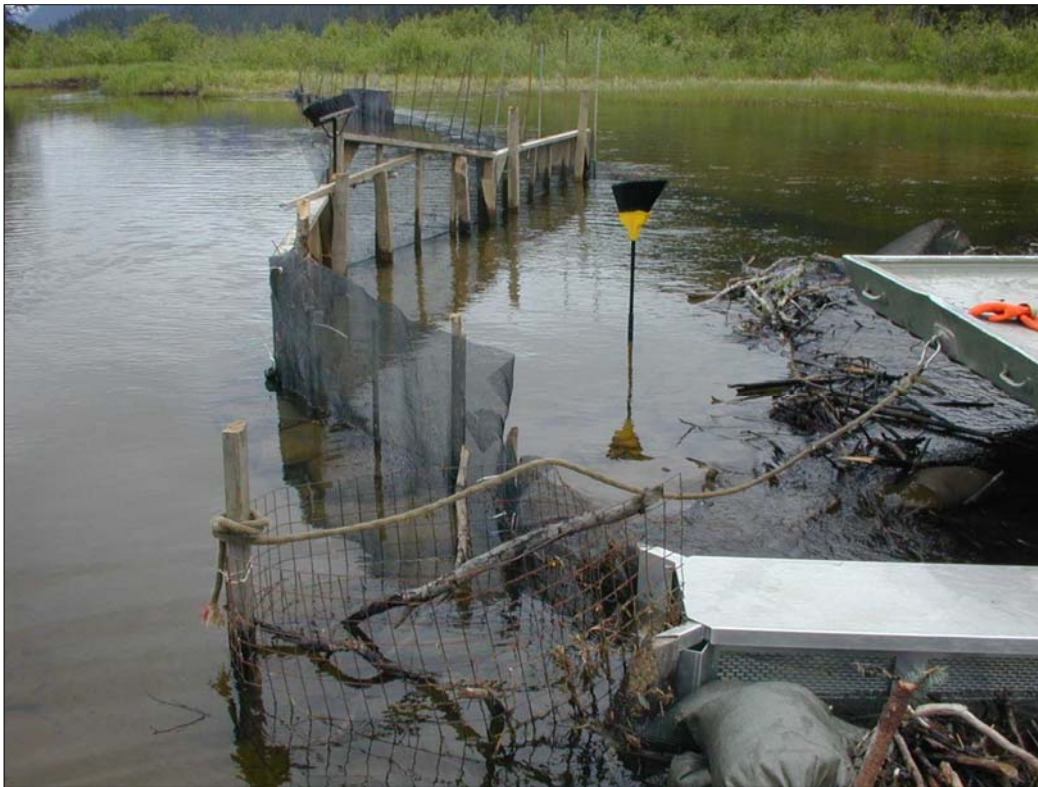
Figure 21. —Water has risen at this spill trap site. A small corral of very sturdy 2-in square mesh wire is installed at the entrance of the trough. This prevents beavers from damming the trough opening. Smolt will readily pass through the large mesh if it is kept clear of debris.
