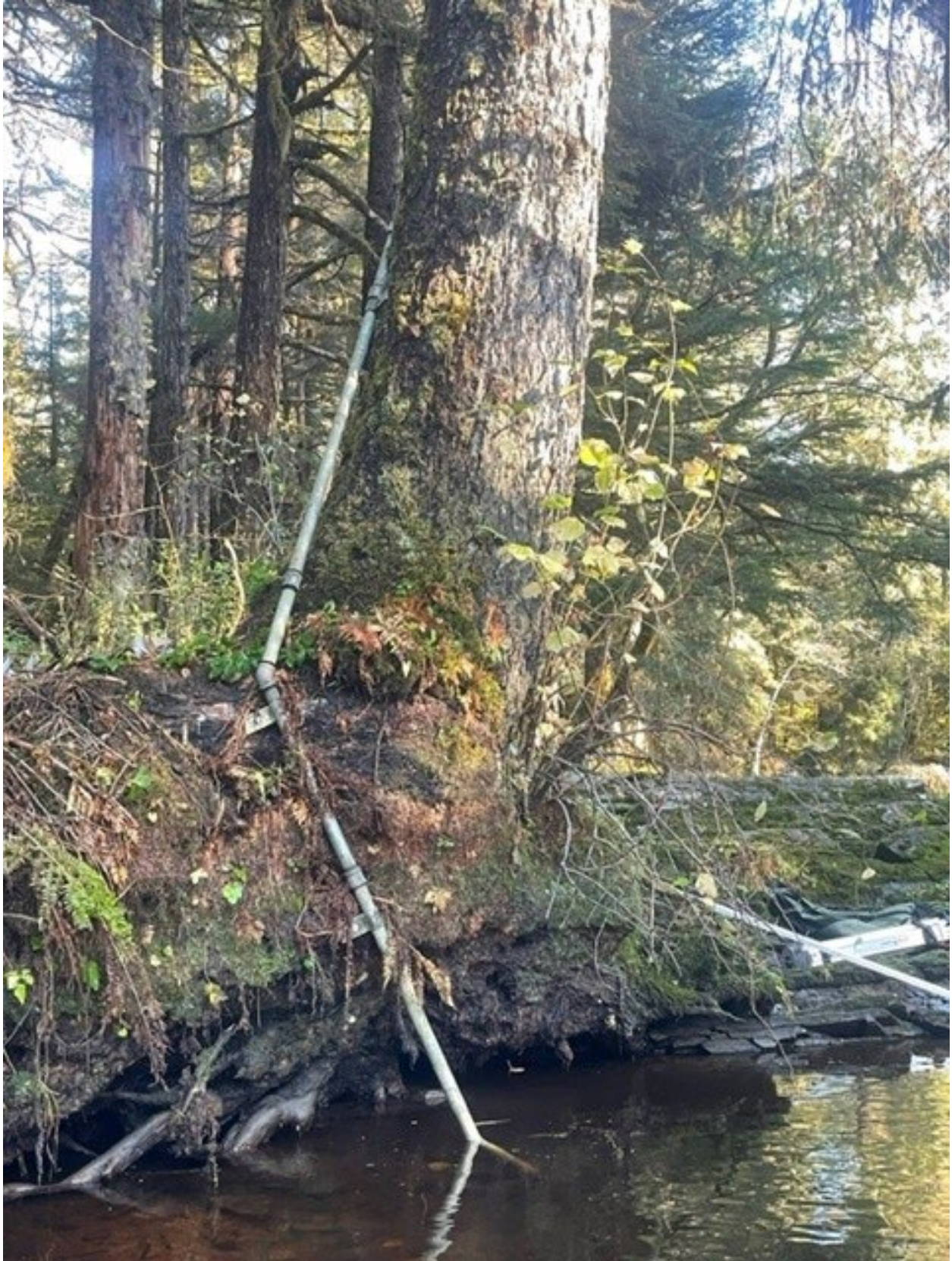
Figure 3.—Salamander Creek Streamgage, after installation on October 6, 2022.
