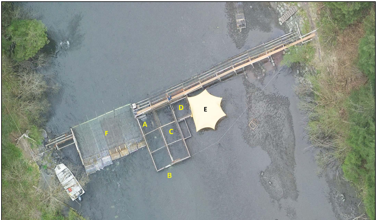
Figure 2.—Overhead view of the Situk River weir and individual components.
