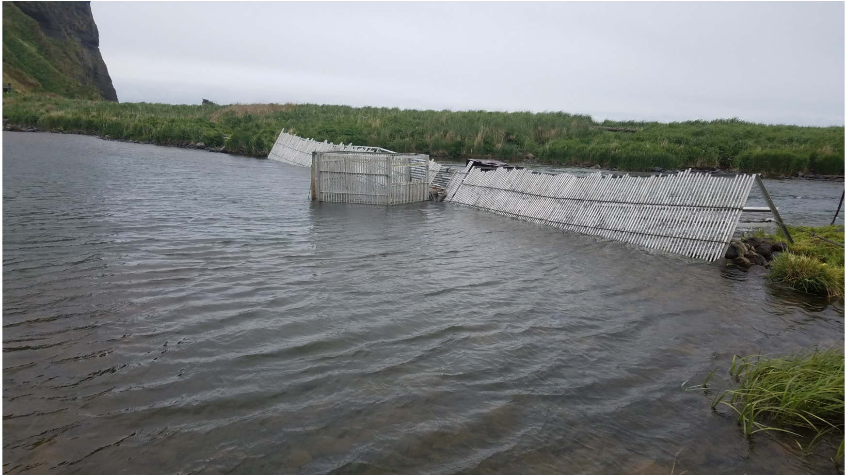
Figure 4.—McLees Lake weir, 2017.
