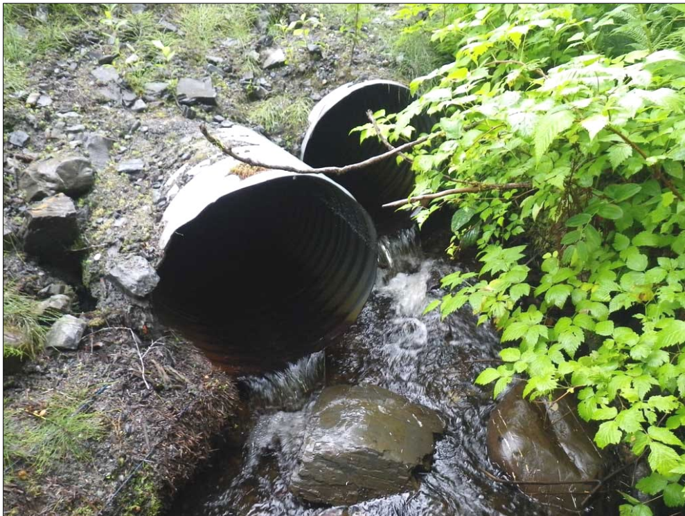
Figure 20.—Site #10302241 in Gustavus showing the Red outfall heights of both culvert outlets. This site also had a Gray constriction ratio of 0.56.
