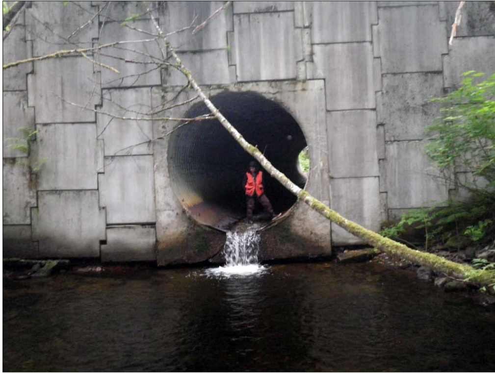
Figure 26.—Site #10302212 on Waydelich Creek off the Glacier Highway in Juneau. Site has a Red outfall, 2.63 ft, and a Red gradient, 2.63%, as well as, a Gray constriction ratio. Stream is cataloged for pink and chum salmon below crossing.
