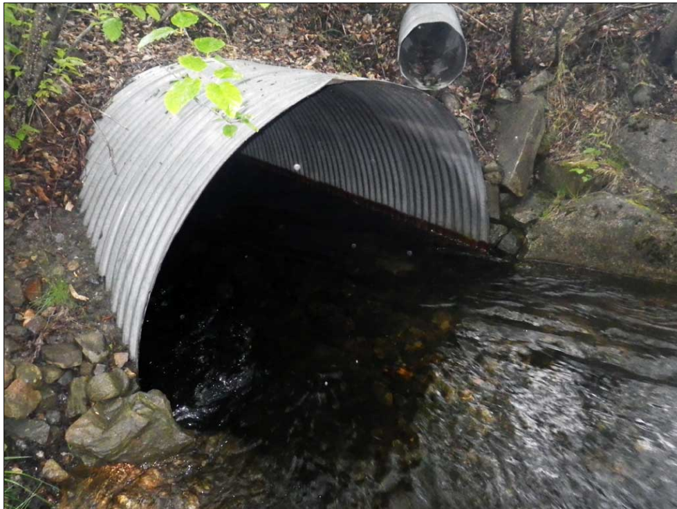
Figure 31.—Site #1030251 with an undersized culvert on Pullen Creek running under Broadway Street.
