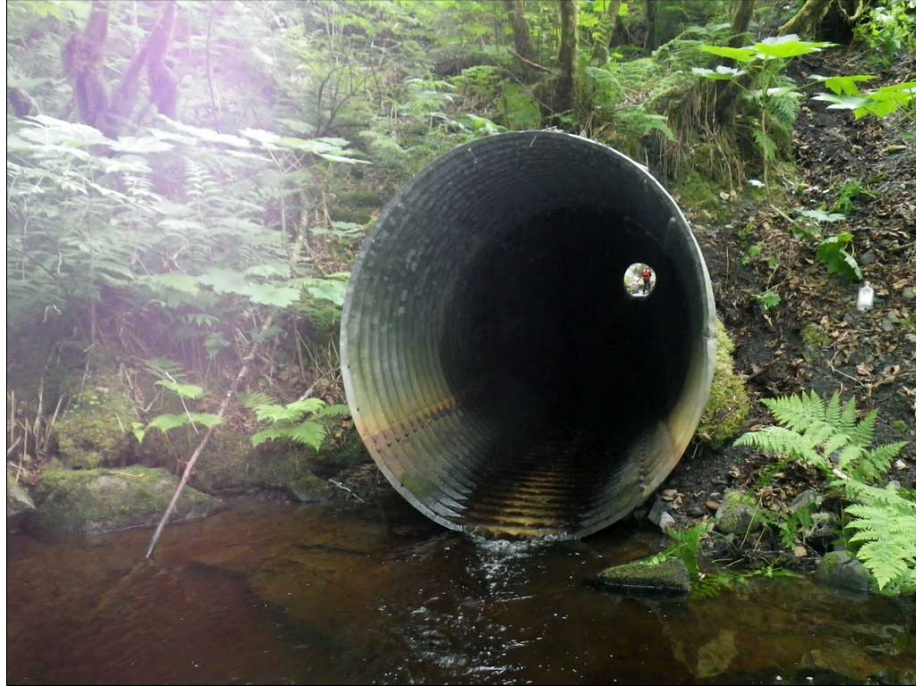
Figure 24.—Site #10302170 culvert on Johnson Creek on the North Douglas Highway. Culvert is Red for gradient and constriction and has a Gray outfall height. Stream is cataloged for coho and pink salmon, Dolly Varden, and cutthroat trout.
