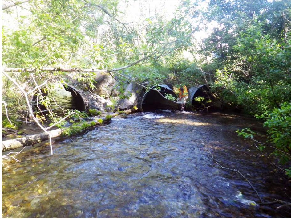
Figure 21.—Site #10302838 on the Porcupine Road north of Haines. The crossing has a Red constriction ratio of 0.40.
