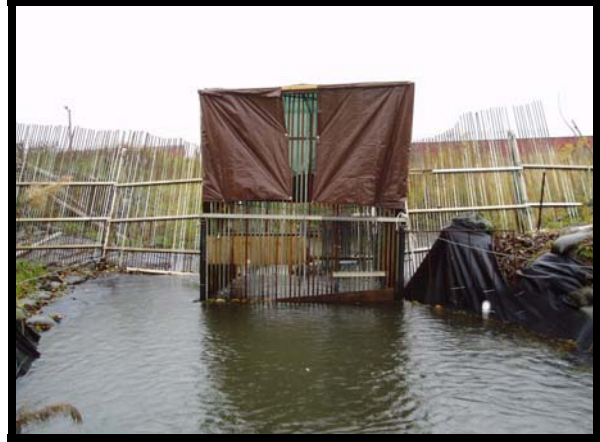
Figure 5.–Downstream view of bipod and picket weir used to capture immigrant fish in Jordan Creek.
