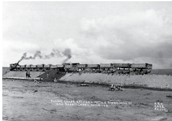
The Alaska Railroad built the Rabbit Creek embankment in 1916-17
