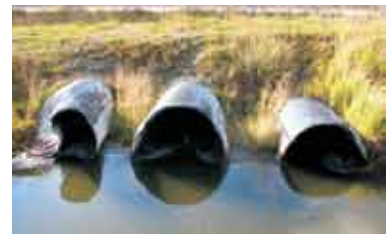
Seward Highway culverts
