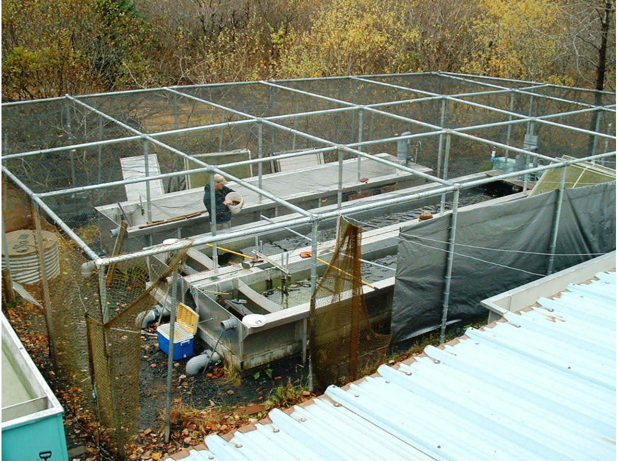
Figure 5. Pillar Creek Hatchery Raceways
