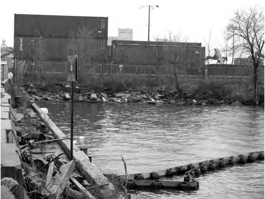
This waterfront property has an abundance of rodent harborage and natural food sources. It is in serious need of housekeeping and vegetation removal to aid in the control of rats and other pests.
