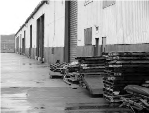
These stacked pallets provide great harborage and concealment for traveling rats tracking along the side of the building.
