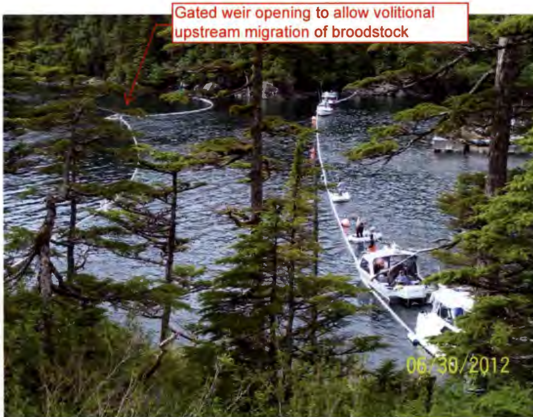
Photo 3: Demonstrated successful use (>15 years) of a cork/buoy-line marker placed seaward of the barrier net weir to preserve functionality and prevent damage and sport fishing inside of the broodstock holding area. The cork/buoy-line marker was removed shortly after this photo was taken as per the request from the Alaska Department of Public Safety based on a complaint that PWSAC was blocking access to an area open to sport fishing.
